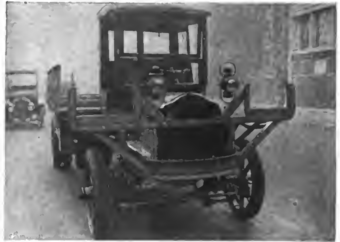
Special body constructed for 5-ton White truck designed for an iron and steel company. Note brackets for extra lengths
